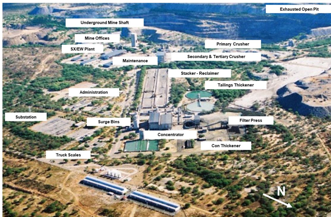
Figure 18-1: Primary Caraíba Mine Infrastructure and Site Layout (Ero Brasil, 2017)
