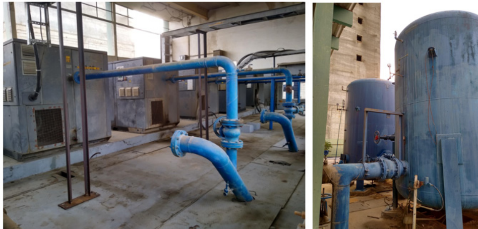
Figure 18-16: Compressed air central station and pressure vessels at surface (Ero Brasil, 2020)
