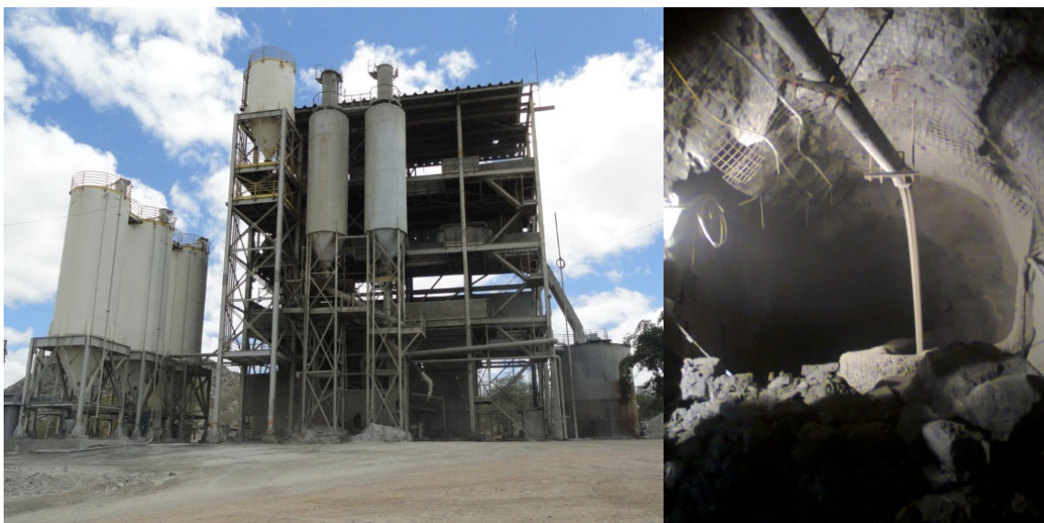
Figure 20-3: Paste fill plant on surface and underground tailings disposal as cemented paste (Ero Brasil, 2022)
