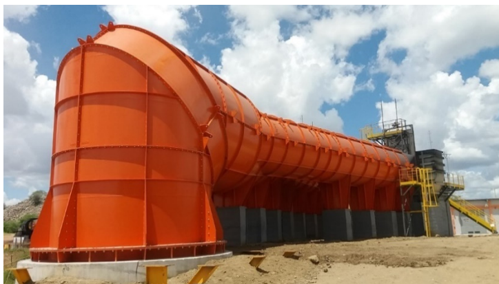
Figure 18-20: P3 exhaust fans – model SOMAX (Ero Brasil, 2020)
