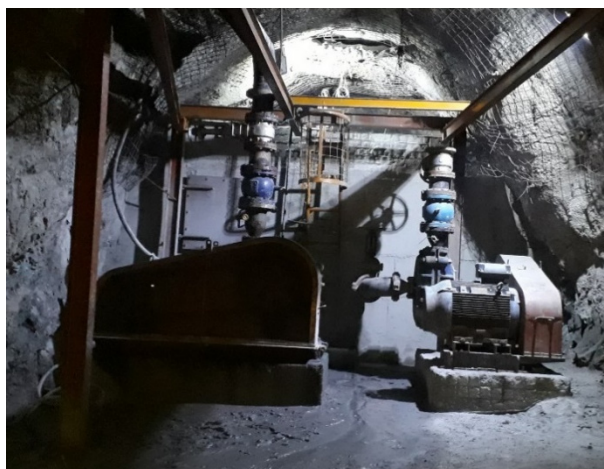
Figure 18-10: Photo of a Main Pumping Station (Ero Brasil, 2020)
